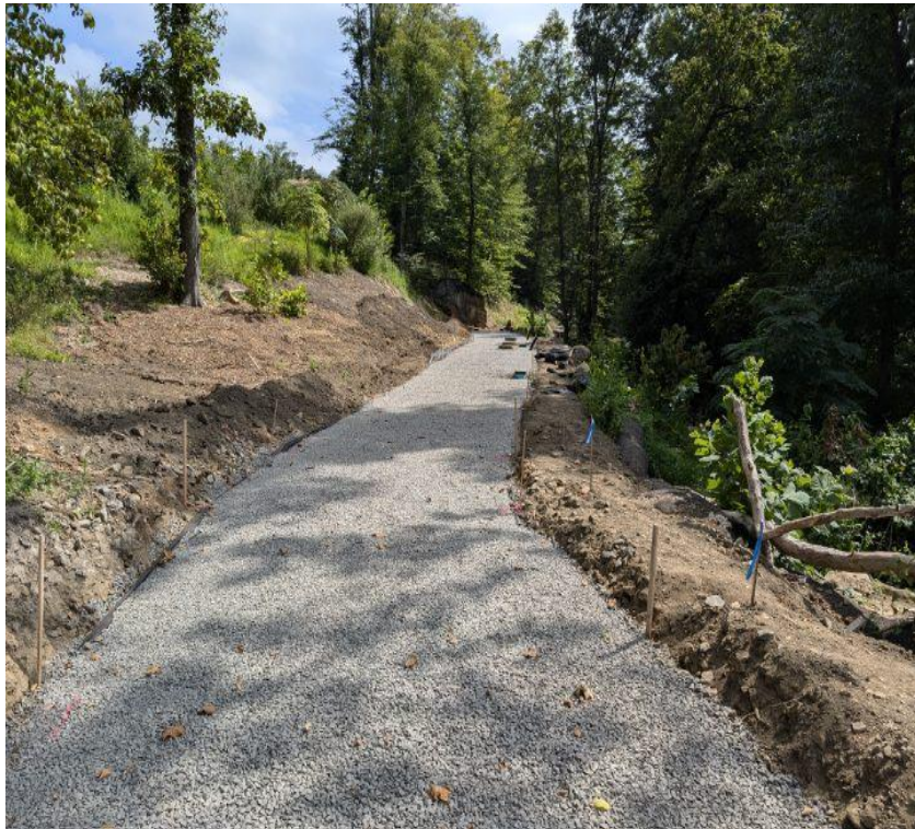
Trail with sub-base
